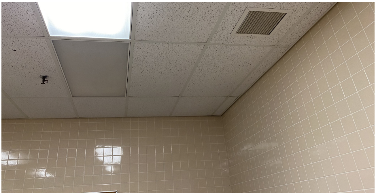
4. Wall to Ceiling Existing Condition
