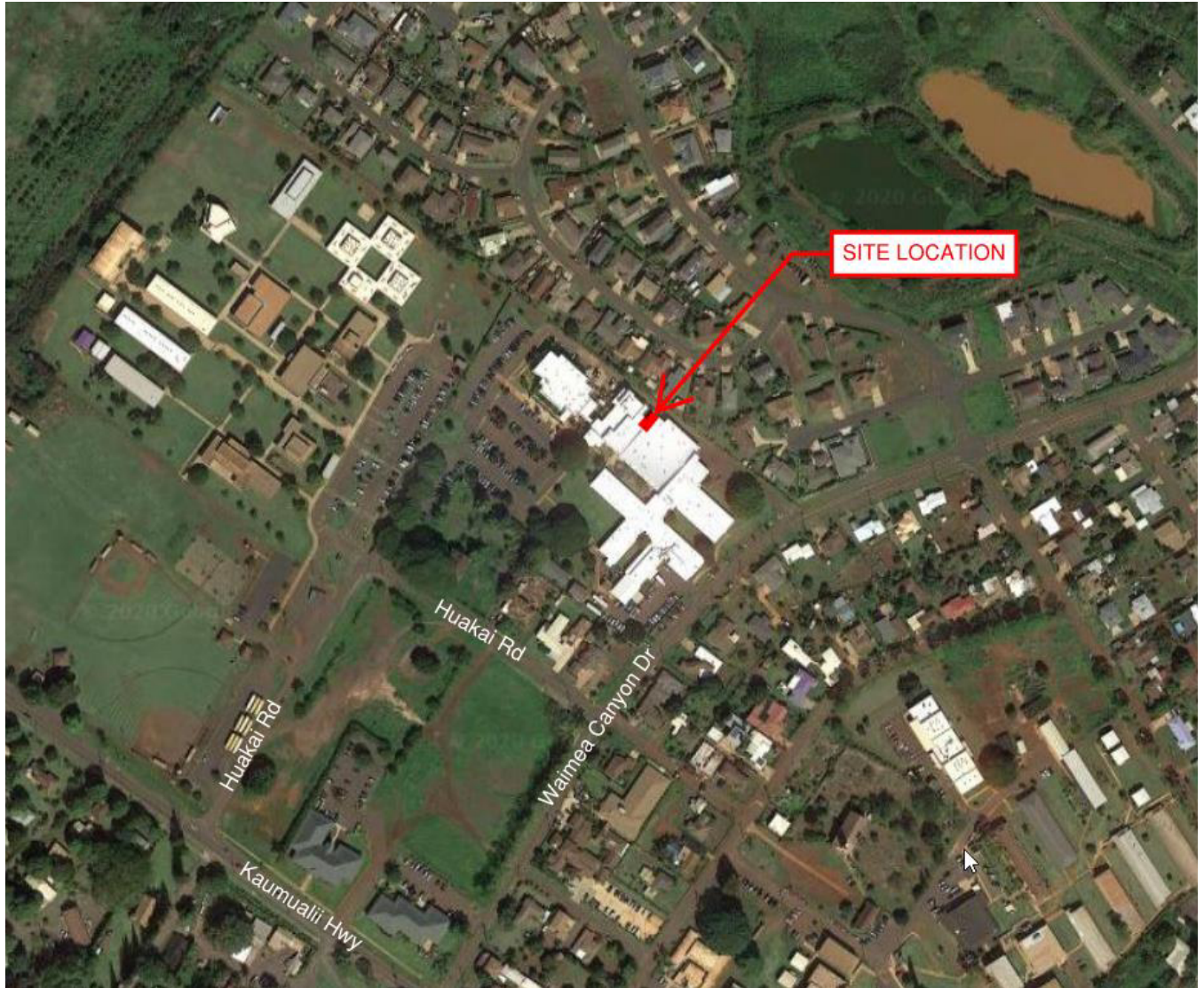
1. Aerial Site Photo
