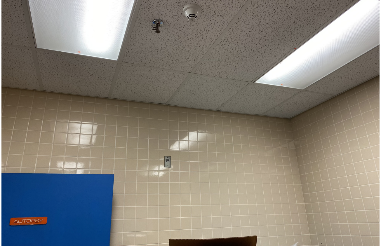
3. Existing Wall to Ceiling Condition
