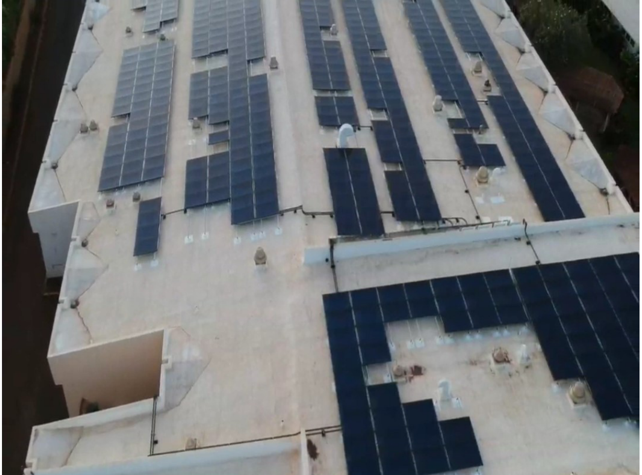
5. Roof Condition at Existing Autopsy Room
